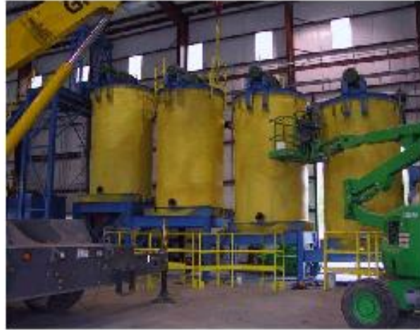
Reactor Tank Installation
