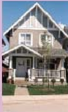
RQ-1 house in the Queensborough neighbourhood, New Westminster
