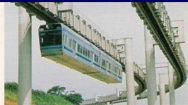
29. Suspended monorail system
