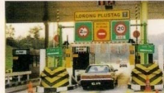
35. Electronic toll collection system
